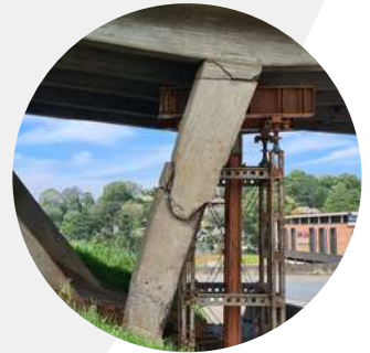
Bridges & bridge jacking
