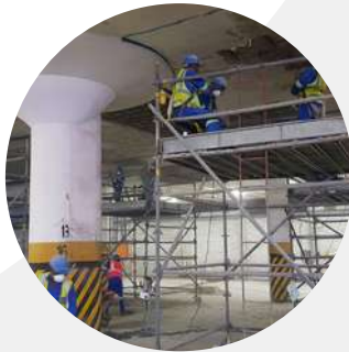
Concrete structural repair
