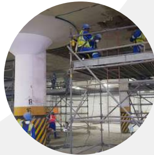
Concrete structural repair
