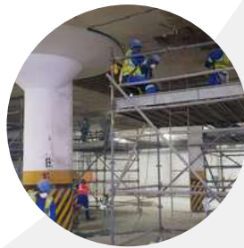
Concrete structural repair
